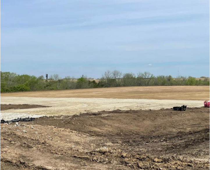
Future Site of new Alliant Energy and ITC Midwest Yaholi Substation near Osceola
