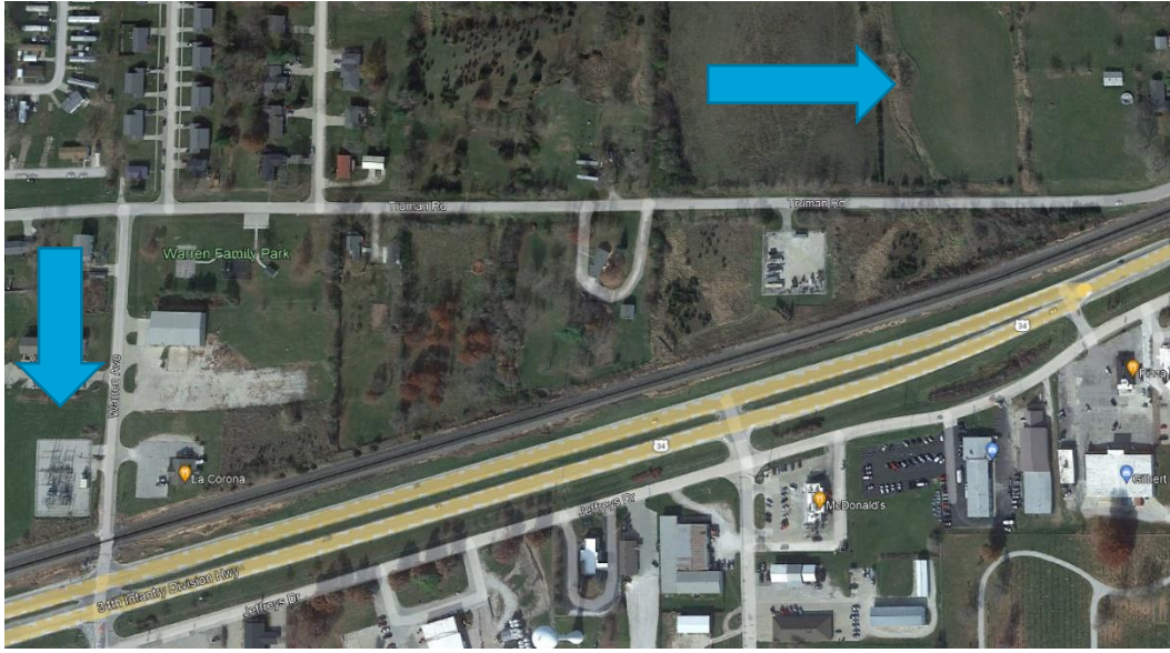
Future site of new Alliant Energy and ITC Midwest Yaholi Substation The existing Alliant Energy Substation will be retired in the future
